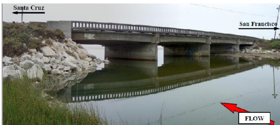
Figure 2.5. Highway 1 Waddell Creek Bridge.
