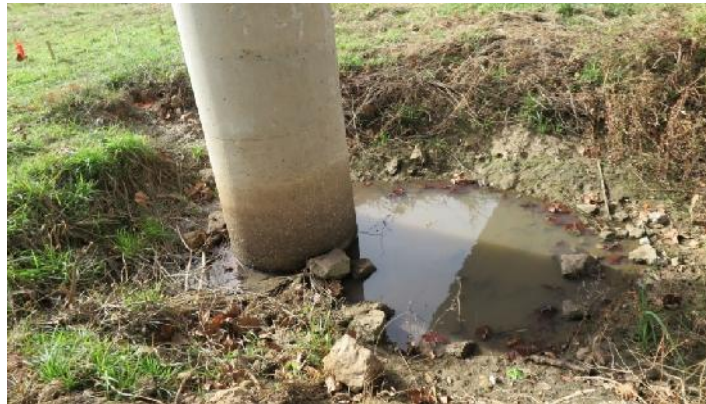
Figure 4.5. The bridge pier with a scour hole as a field test site.
